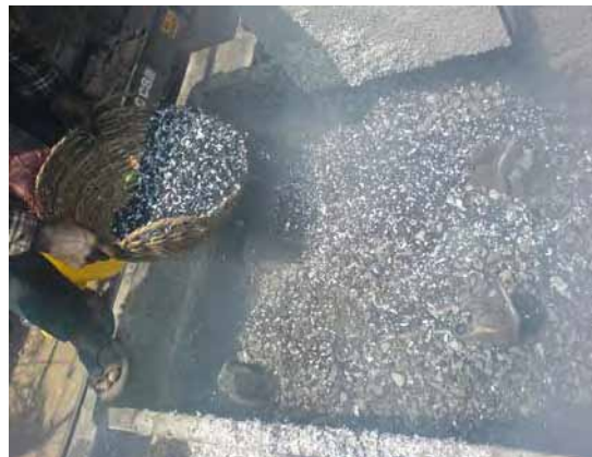
Plate 2 Preparation of plastic coated aggregates (PCA) in the field
