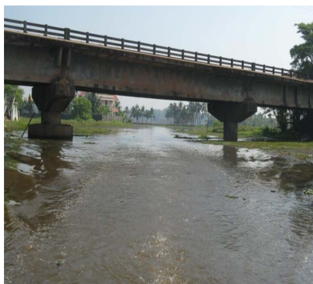
Plate 11 Manakkakadavu Road Bridge
