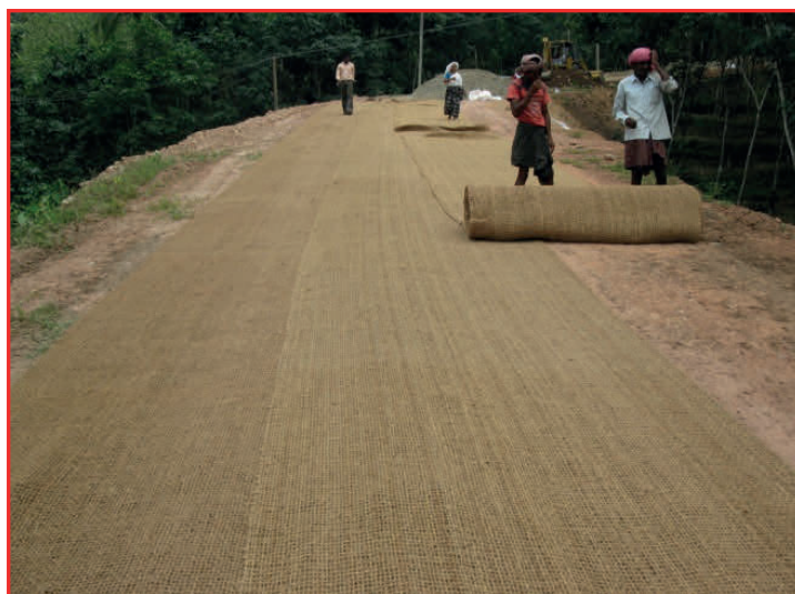
Plate 8: Laying of Coir geotextiles along Karikkuri - Chekidampara Road
