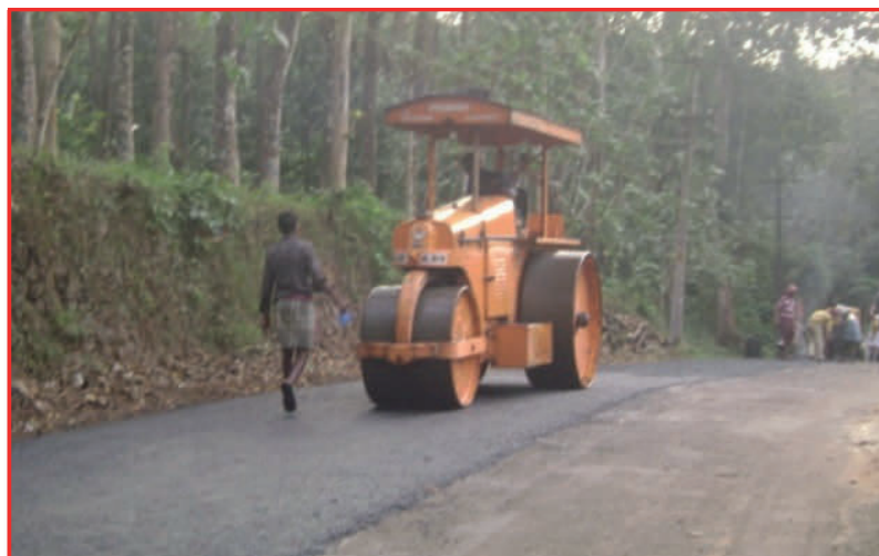
Plate 4 Laying of plastic road in Mutholi-Poovar ani Road
