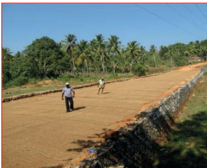
Plate 7: Laying of Coir geotextile along Njekkadu-Panayara Road
